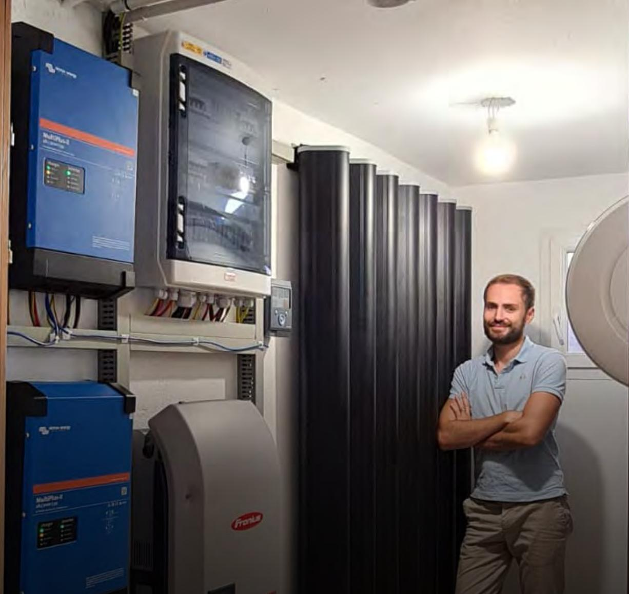
Systeme Studer 8 Kva 1ph / Victron 9kVA tri-phase
